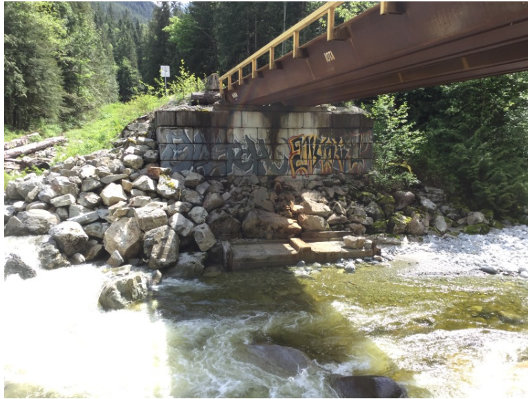
Left Bank Abutment when facing downstream
