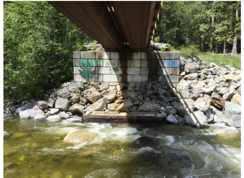
Right Bank Abutment when facing downstream
